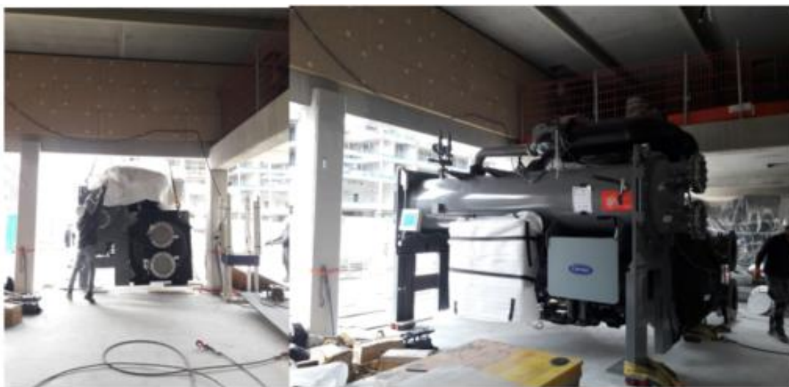
Figure 58 : Heating and cooling production systems implementation (Source: MSE)
