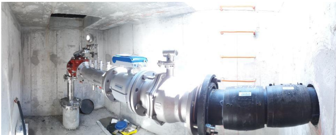
Figure 59 : He Geothermal well chamber (Source: MSE)
