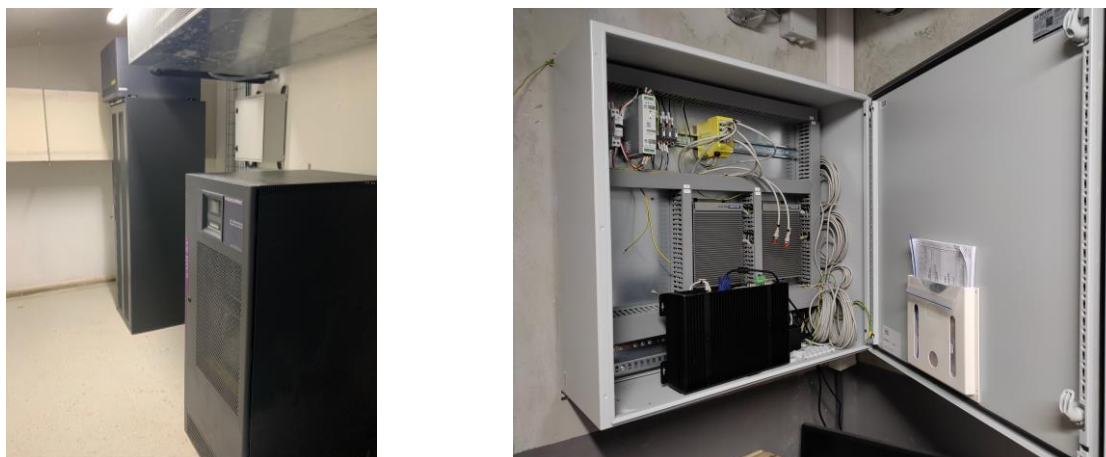
Figure 13 : Battery storage system and the EMS in the PALAZZO building
