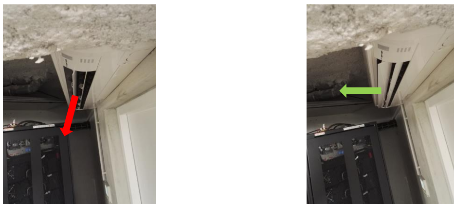
Figure 41 : Left /Air conditioning blowing directly on the battery – Right/Correct position
