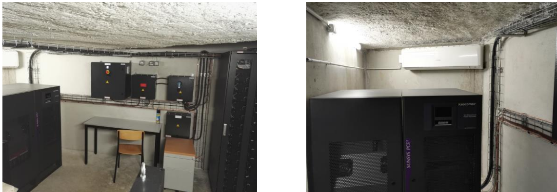
Figure 9 : Lithium-ion battery system at IMREDD.
