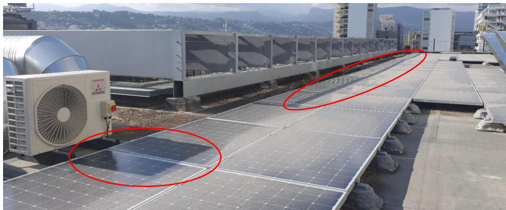
Figure 27 : Example of shadings on the photovoltaic panels of the IMREDD building
