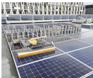
Figure 32 : Cleaning of the photovoltaic panels
