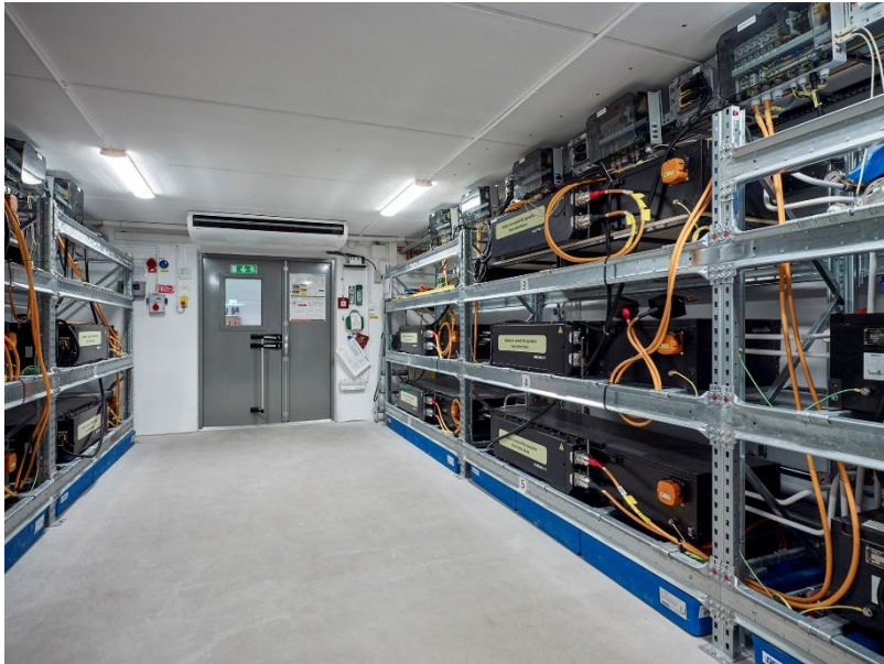
Figure 8 Inside the battery storage room.
