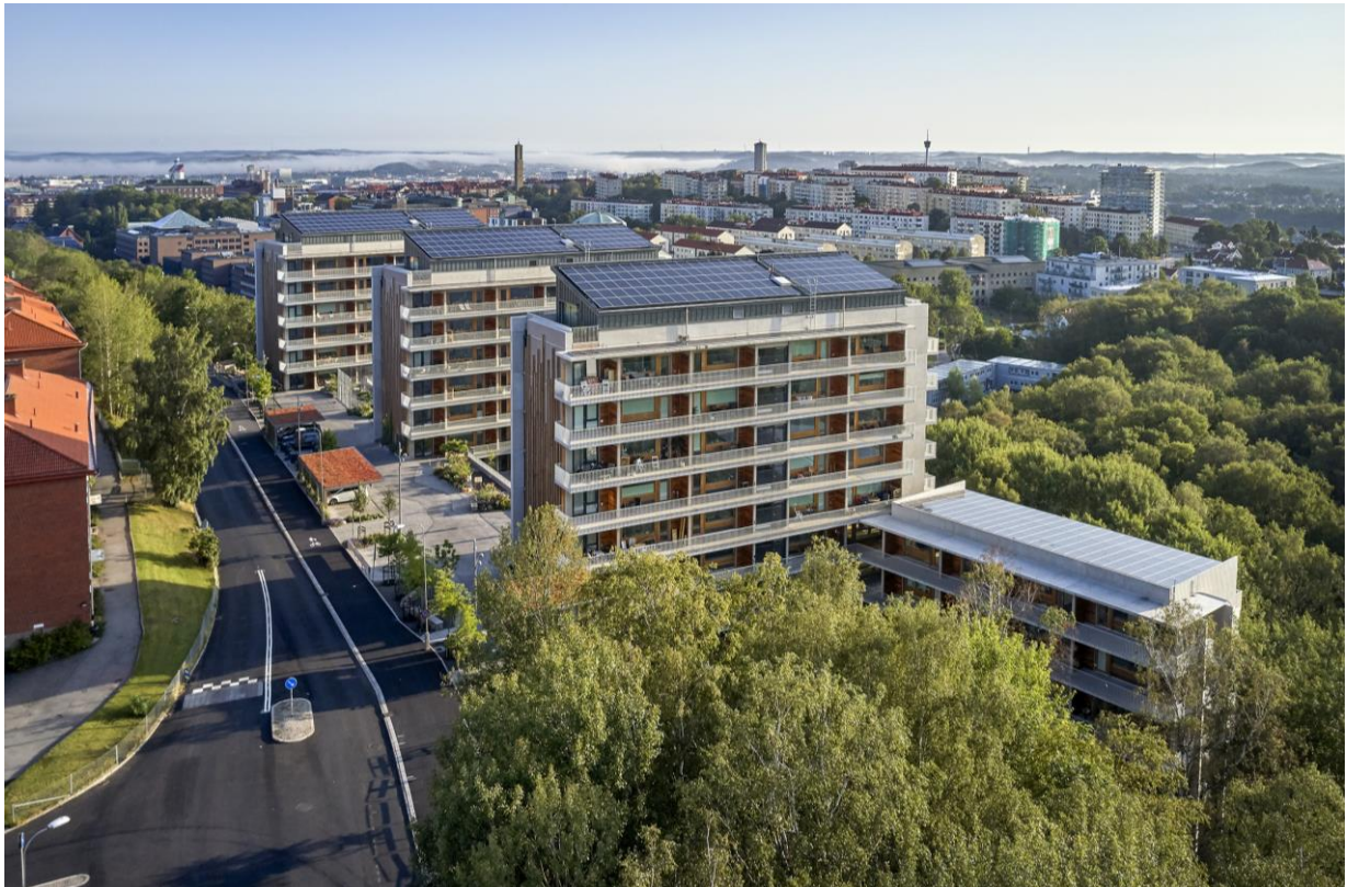
Figure 12 Brf Viva with its PV clad roofs
