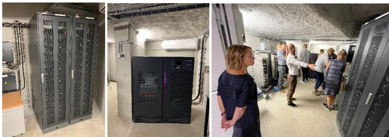
Figure 117 : from left to right – IMREDD's two battery stacks, inverter, and view on the overall BESS room. (source: EDF)
