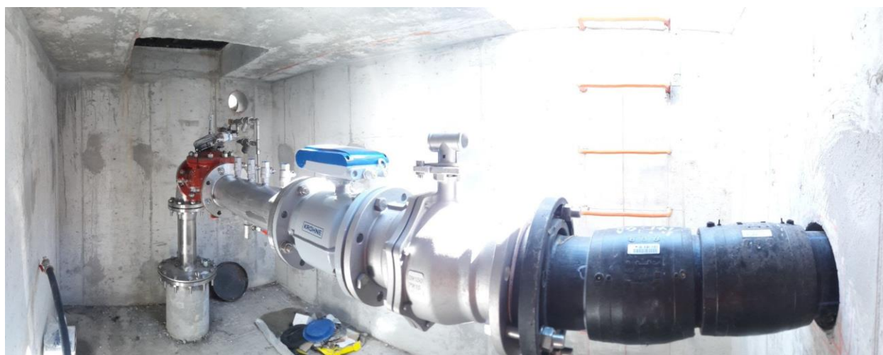
Figure 105 - Geothermal well chamber
