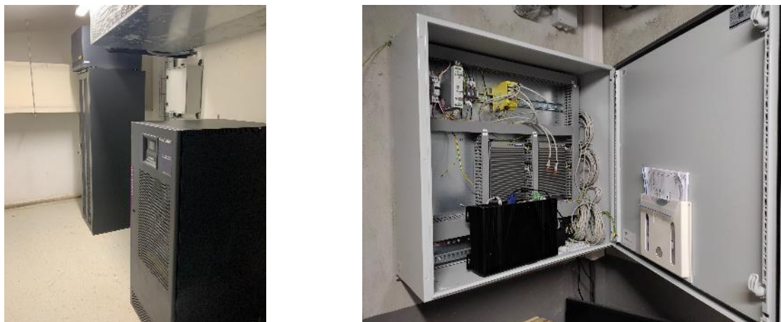
Figure 16 : Battery storage system and the EMS in the PALAZZO building
