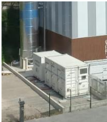
Containers housing the battery and his power converter
