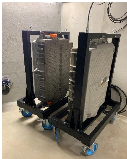
Figure 116 : IS 2.3, 2 nd life batteries from Renault Kangoo – system ready to be connected to the BEMS and inverter (Source: EDF)
