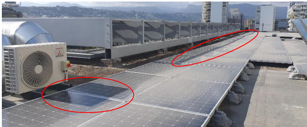
Figure 83 : Example of shadings on the photovoltaic panels of the IMREDD building
