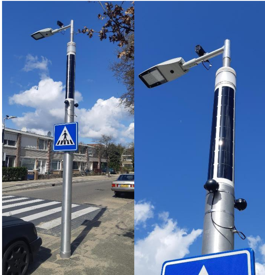
Figure 27: luminous smart pedestrian crossing and smart poles
