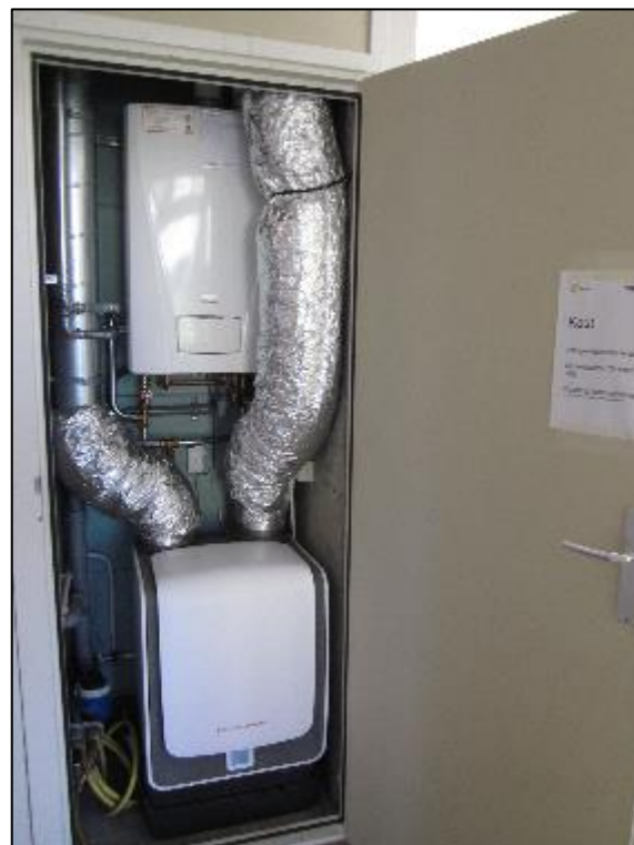
Figure 7 Eneco Warmtewinner heat pump icw gas heated boiler (Bo-Ex)
