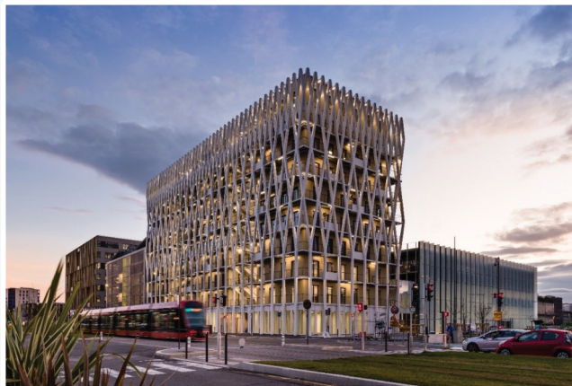
Figure 3: Palazzo Meridia building and the IMREDD building on the right hand side. (Source: © Y. Bouvier for Nexity)
